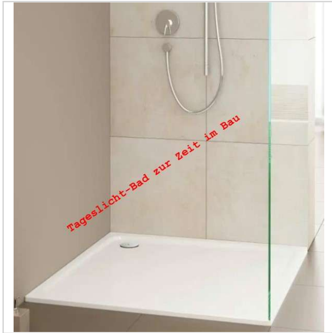
Bad in Bau
